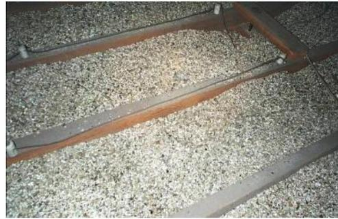
Largely, the non-asbestos vermiculite attic insulation comes from South Africa. This is somewhat larger in size than Zonolite. There were also attic insulation products sold that included a mix of Zonolite and South African Vermiculite.
